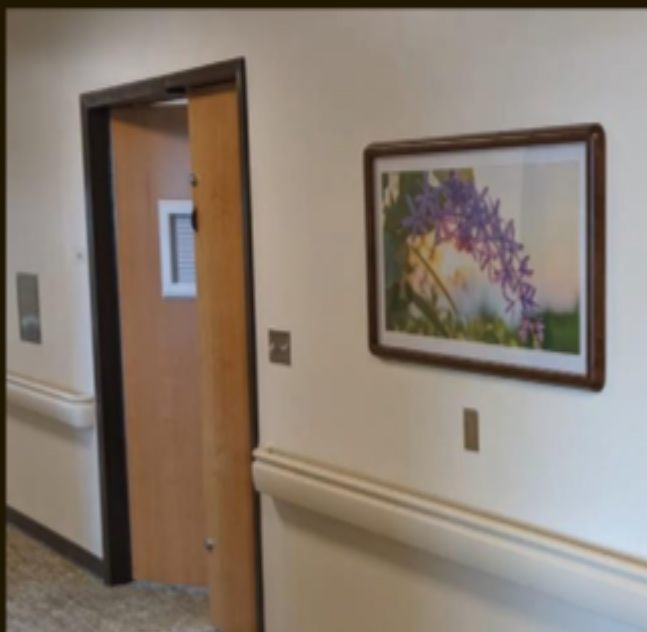
Compound radius corners eliminate sharp edges and are ligature resistant.
